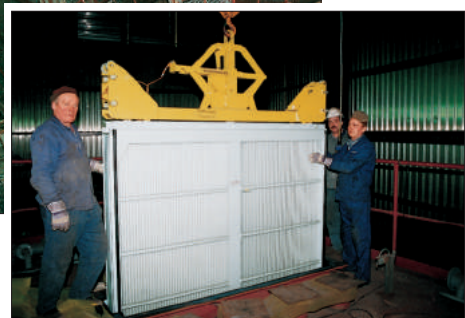
LTH 100 beeing installed in a flue-gas desulphurization plant
