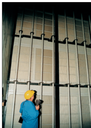
Installed LTH 100 in a flue-gas desulphurization plant
