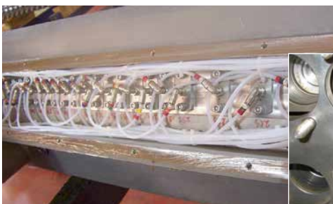
Pneumatic header after refurbishment
