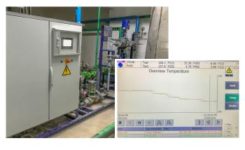
VarioCool® valve skid unit with SmartControl software
